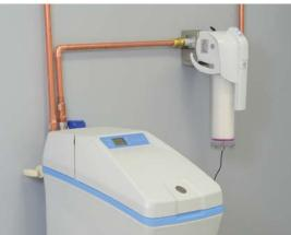
Whole home filtration connects to your home's main water line to reduce sediment, scale, dirt and rust.
